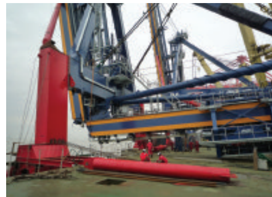
Positioning the cranes on deck with special support
