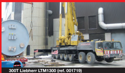
300T Liebherr LTM1300 (ref. 001719)
