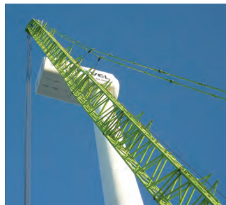
Nordic Crane at work in Molkom, Sweden, with a Liebherr LG 1750 and 105 metre boom
