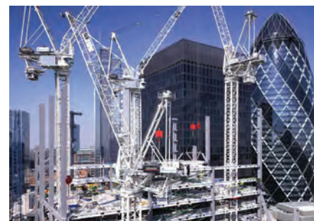
Still operated in free standing mode the Terex luffers overlook the first levels of the Leadenhall Building surrounded by the prominent London inner city skyline. In the front of the photo the short 30 m boom of the CTL630-32, a tribute to the cramped site conditions, can be seen
