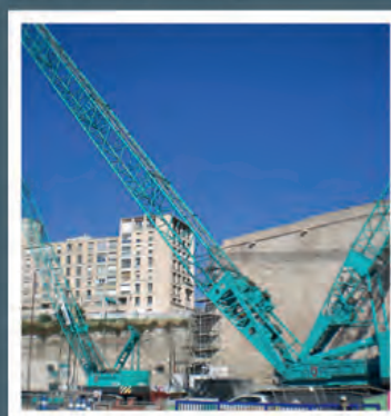
Kobelco SL6000, 550 ton capacity
