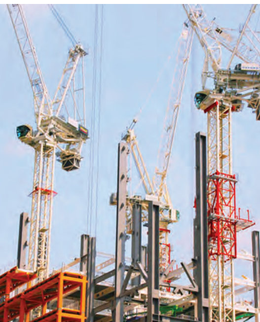
While the crane on the left of the picture is jumped as an internal climbing crane, the two on the right still have a climbing cage for external climbing
