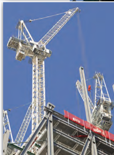
The Terex CTL630-32, left, needs extra ballast at the rear of its machinery deck when it is being operated with a shortened boom. The new CTL650-F45 on the right can be installed with just its standard movable ballast in short boom configuration
