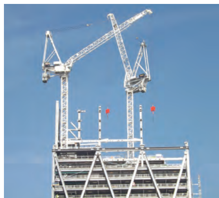
The two remaining Terex tower cranes on top of the almost-finished Cheesegrater building in the City of London, March 2013
