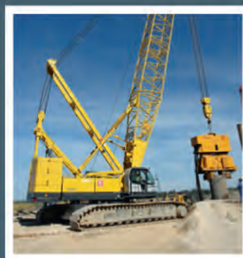
Kobelco CKE2500, 250 ton capacity
