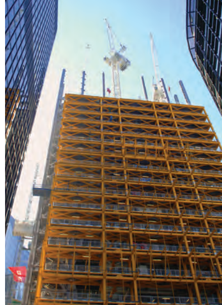
The yellow service core on the north side of the building made up of table-like 35 tonne modules installed by the two CTL650-F45 luffing jib tower cranes
