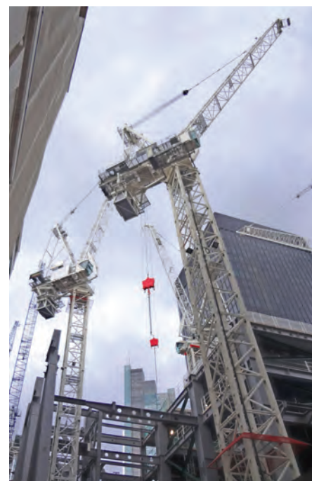
The two CTL650-F45 and one CTL630-32 Terex luffing jib tower cranes in their initial phase of the Leadenhall Building construction process
