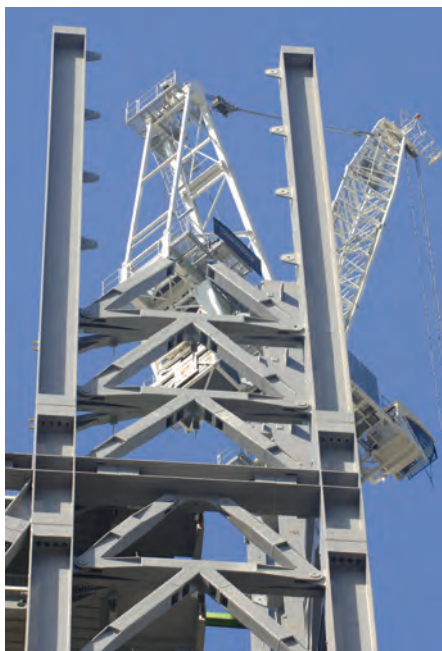
Up to 28 m high mega frame columns have to be installed. Using internal climbing luffing jib cranes means jacking can be delayed by raising the boom and using the 48 m free standing capacity
