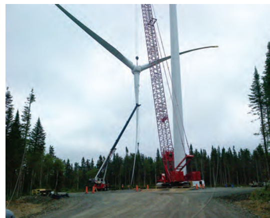
A Manitowoc 16000 crawler crane on a job site in Northern Quebec, Canada
