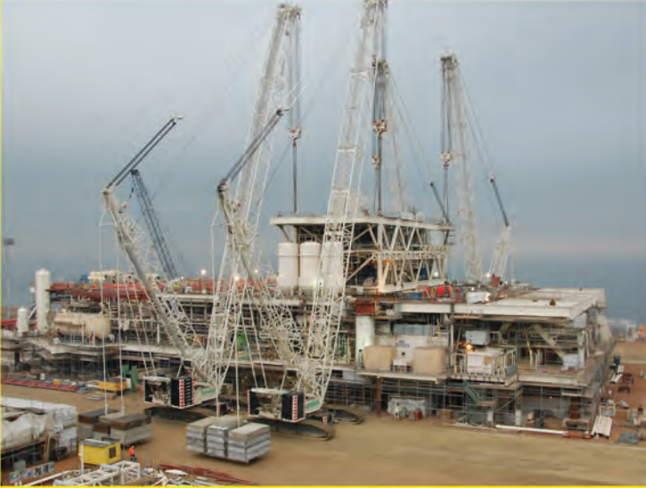
Erection of 1126 tons DSM module by 4 units of Demag CC 2800-1 in Chirag Oil Project Baku, Azerbaijan constructed by Amec-Tekfen-Azfen consortium for BP.
