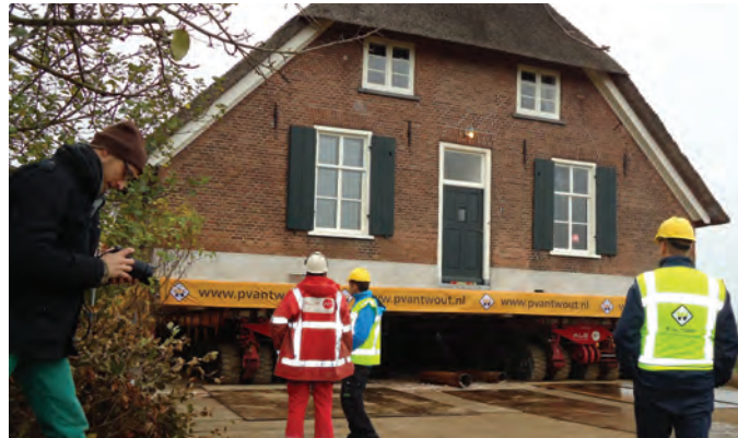
The farmhouse being transported on SPMT
