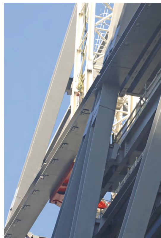
Based on careful 3-D planning a solution was found to base the climbing crane on a special lower climbing collar before leaving the tapering shaped front of the building under construction
