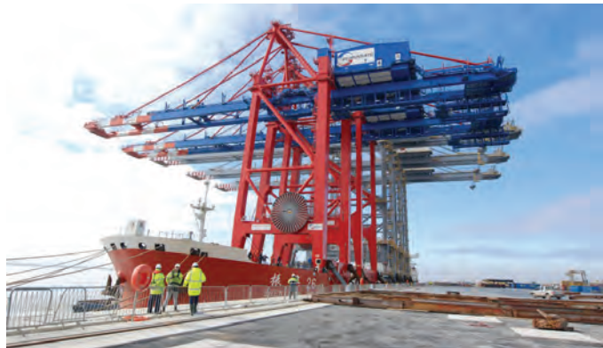
The cranes on the quay of the DP World London Gateway, the UK's new global shipping port
