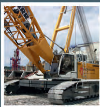
Liebherr LR1300, 300 ton capacity
