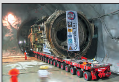
Bridge & Tunnel Construction
