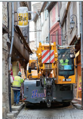
The mobile crane carefully worked its way through the sleepy mediaeval town in the early morning
