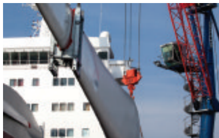
A mobile harbour crane lifts a Vestas tower section
