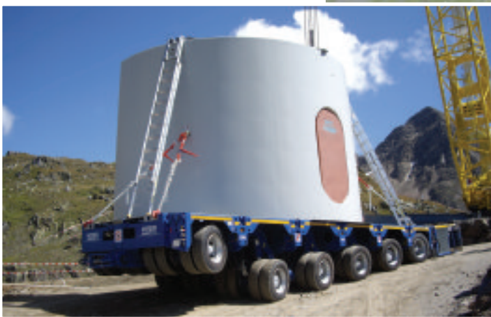
Arrival of the 40 tonne half-shell section of the concrete tower. The first axle line was lifted to achieve better traction when transporting a low load
