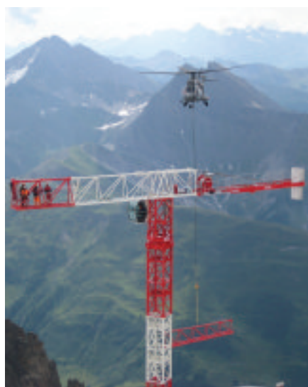
Several helicopters were hired to help assemble the two Saez tower cranes for the Cordée Mont Blanc group
