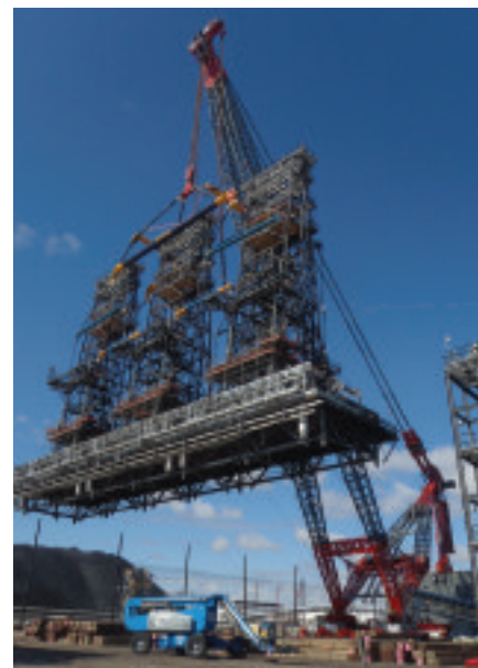
The AL.SK190 with complex 12-point rigging arrangement working at the Valero refinery in Texas, USA, earlier this year. For the full story see IC September 2011, page 16.
