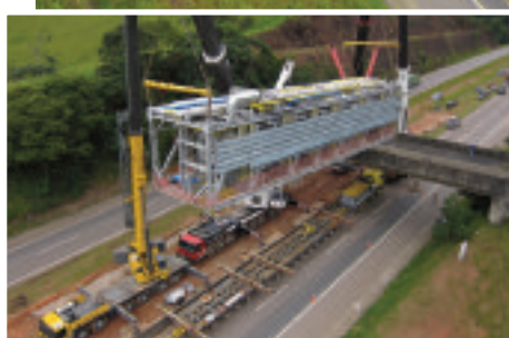
A section of a footbridge is raised using hydraulic gantries to allow the transport to continue on its journey
