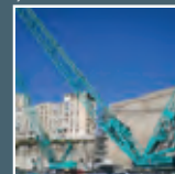
KOBELCO SL6000, 550 ton capacity
