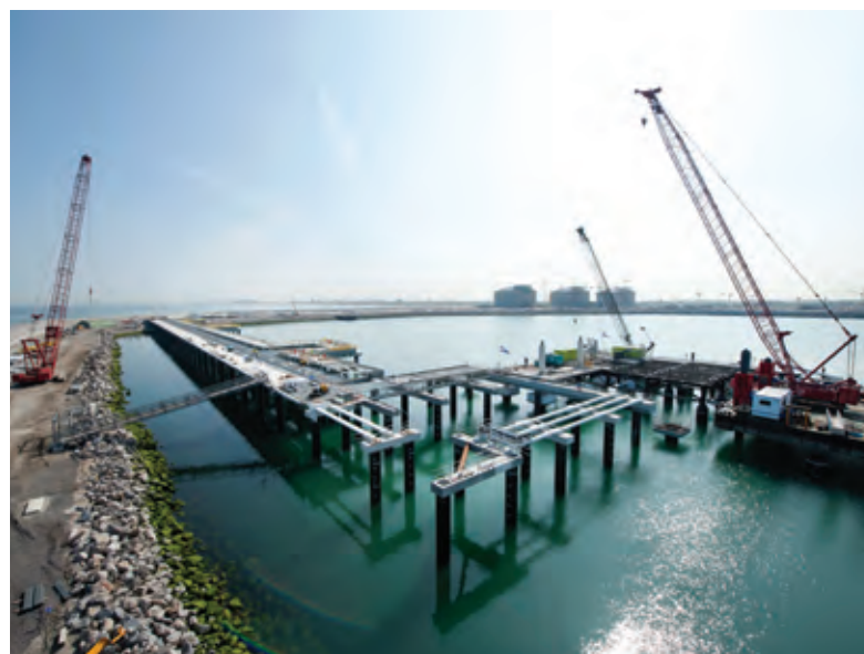
Recent work for the crawler cranes in Dunkirk has included constructing a terminal jetty
