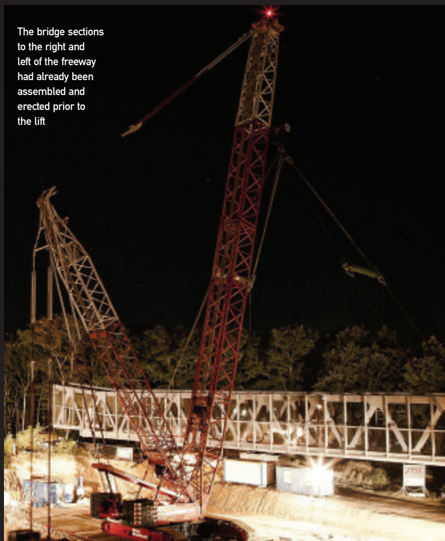
The CC 2500-1 puts the 70 metre-long steel footbridge in place
