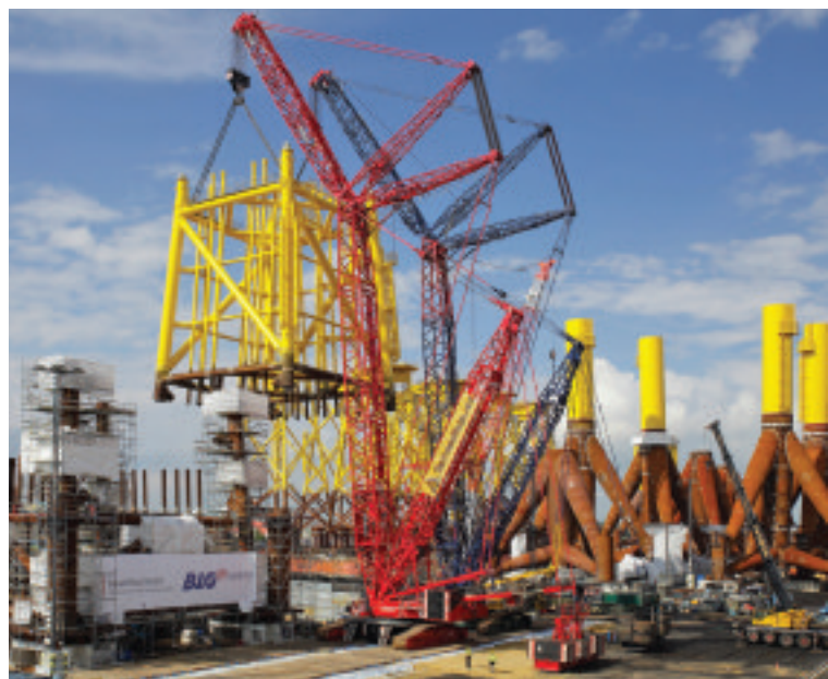
Two Liebherr LR 1750 crawler cranes work in tandem to lift a 600 tonne jacket structure at the ABC-Halbinsel offshore terminal in Bremerhaven
