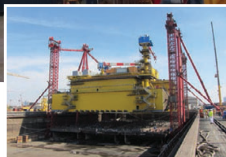
ALE prepares to lift the world's first semi-submersible HVDC platform, the DolWin Beta
