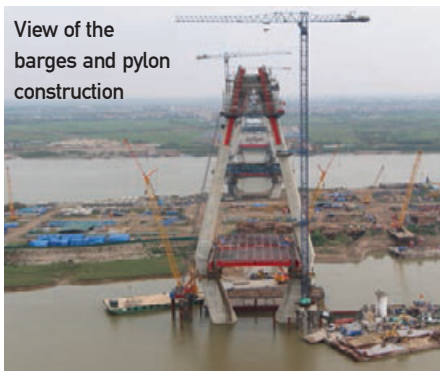
The additional foundations increased the cranes' height by between 5 and 11 m
