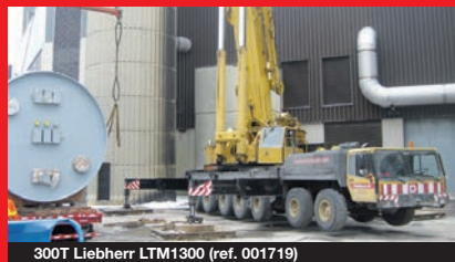
300T Liebherr LTM1300 (ref. 001719)
