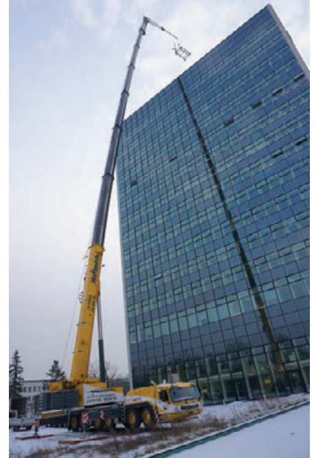
Manitowoc's 400 tonne capacity Grove GMK6400 all terrain
