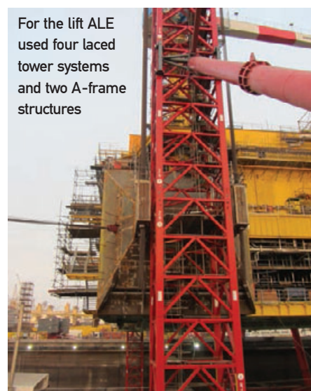
ALE prepares to lift the world's first semi-submersible HVDC platform, the DolWin Beta
