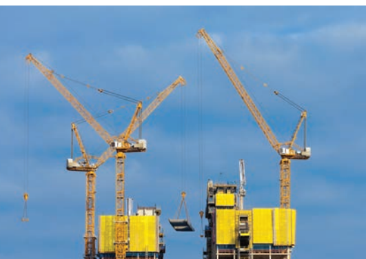
Liebherr's 542 HC-L tower crane is designed with large 110 kW winches for fast and powerful hoisting and luffing
