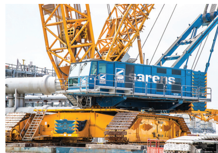
The crawler's two 14.4 metre long and 2 m wide tracks helped spread the load
