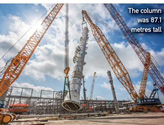
After this lift was completed with the Boom Booster the the Terex CC 8800-1 was dismantled and shipped back to Sarens' yard
