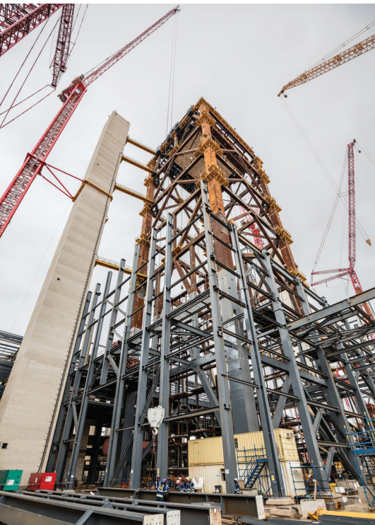
The Wolff 1250 B with a 60 metre jib and a tower height of 120 m is tied to the stair tower of the boiler house with just one tie
