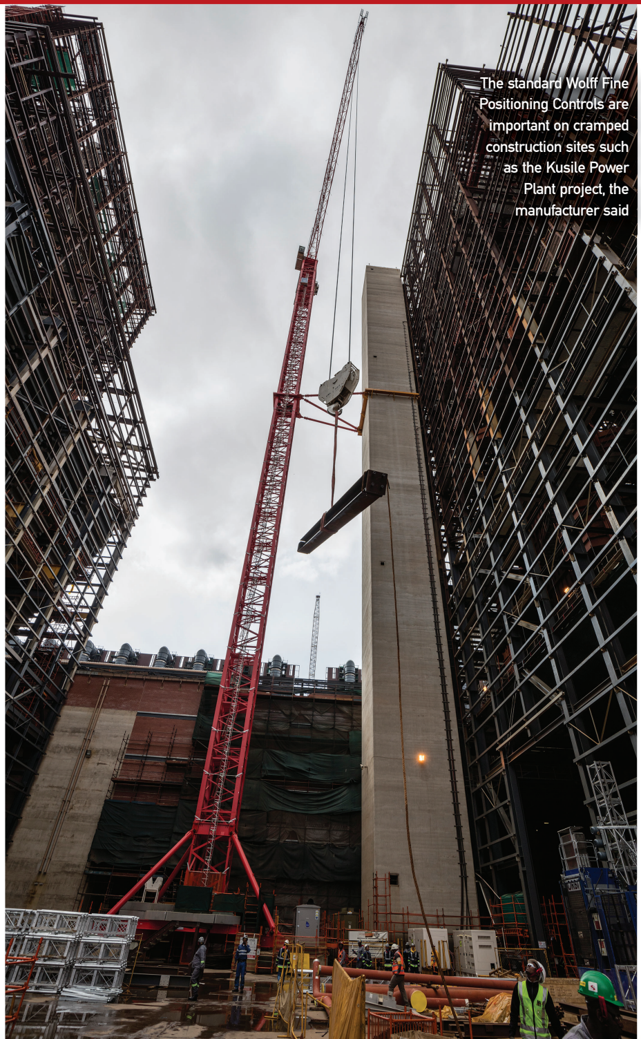
The Wolff 1250 B with a 60 metre jib and a tower height of 120 m is tied to the stair tower of the boiler house with just one tie
