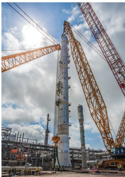
After this lift was completed with the Boom Booster the the Terex CC 8800-1 was dismantled and shipped back to Sarens' yard
