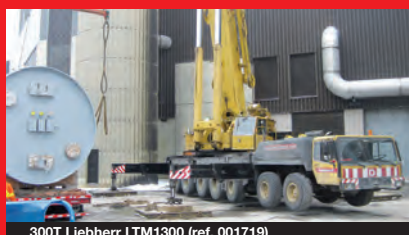
300T Liebherr LTM1300 (ref. 001719)
