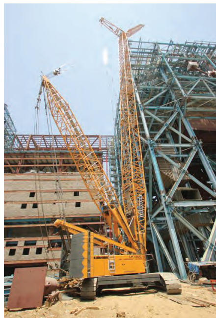
A Liebherr LR 1300 crawler crane at the Koradi Thermal Power Station expansion project close to Nagpur in Maharashtra, India
