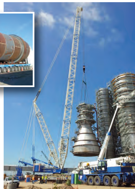
Roll-Lift working on the Montes Del Plata project with Andritz Pulp & Paper a Finnish company in Uruguay
