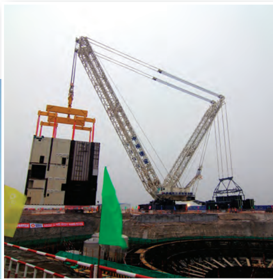
A Terex CC 8800-1 Twin at work at a project in China
