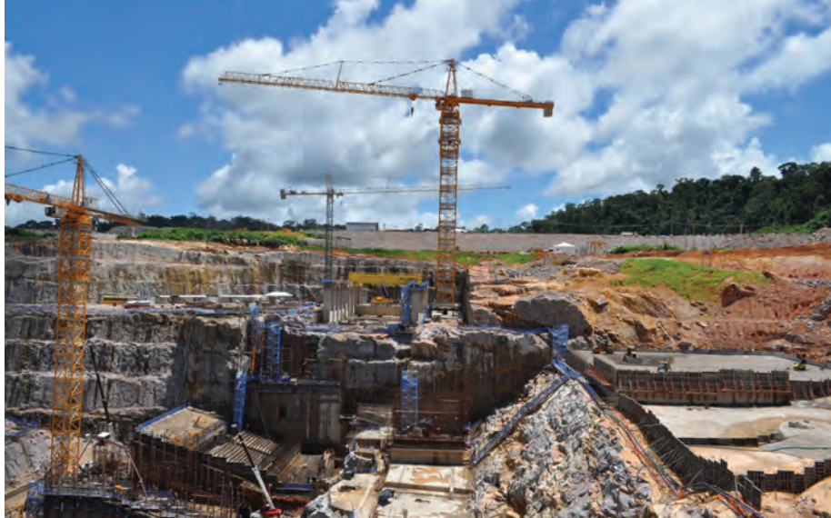
A Liebherr 2000 HC 60 and a 1250 HC 50 tower crane in operation on the construction of the Teles Pires hydroelectric plant, in Mato Grosso
