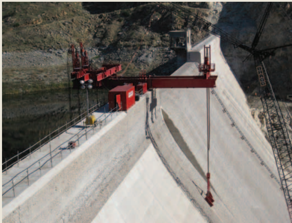
Barnhart engineered a cantilever system to carry out Cofferdam section lifts
