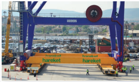
Two 28.5 m beams were put on the trailers to help transfer the weight of the crane
