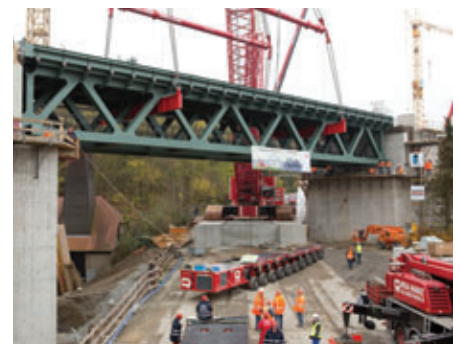
Positioning the 355 tonne load precisely on the abutments of the future railway bridge
