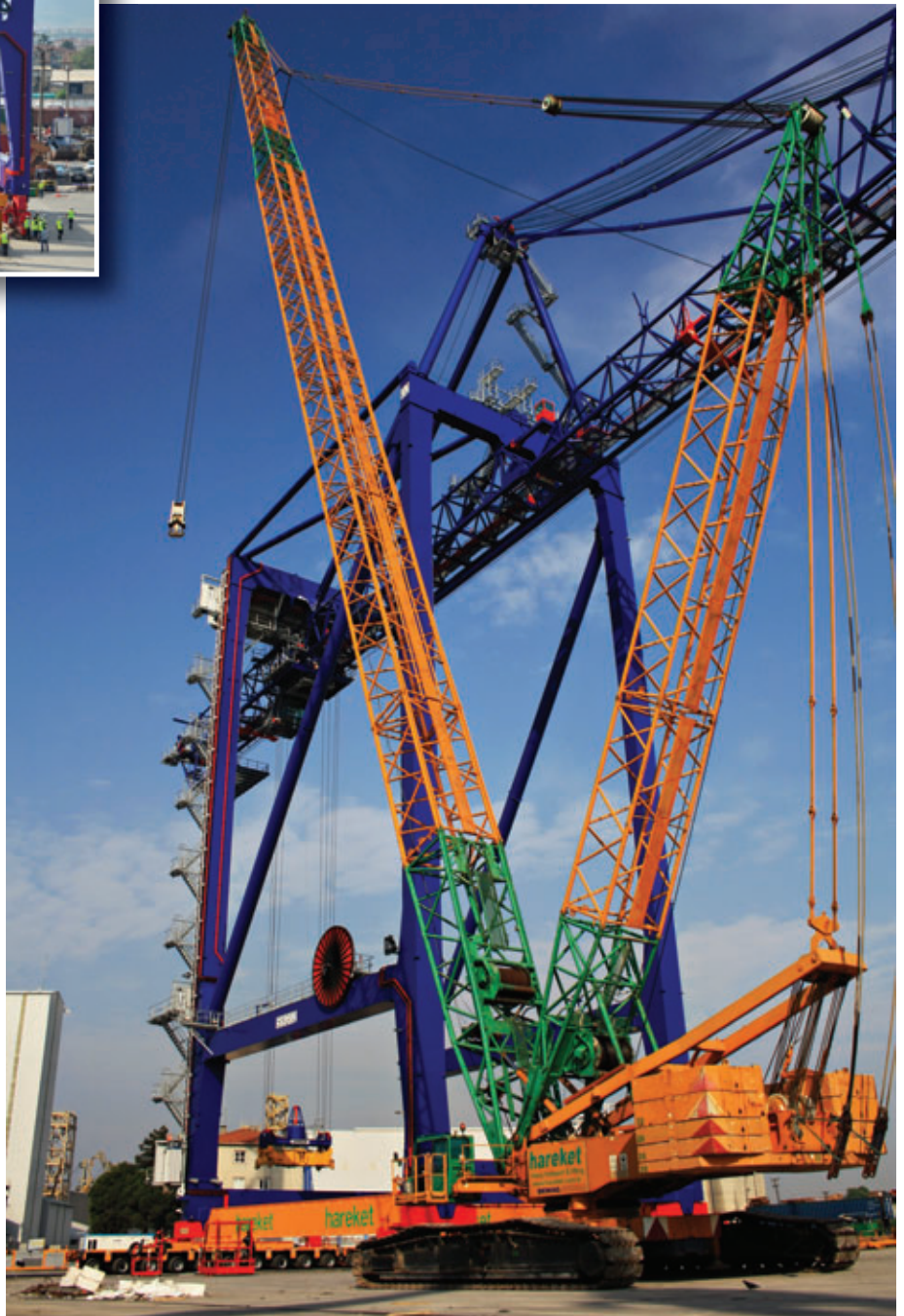
The cranes arrived at Derince port by vessel in sections and were assembled by the port's mechanical and electrical contractor Portunus
