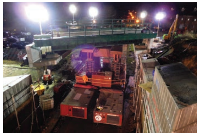
ALE jacking the Cleatham Road bridge in Lindsey, Lincolnshire, UK
