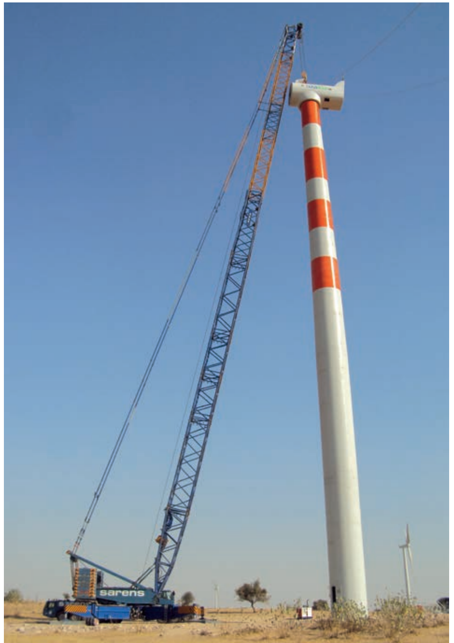
A Sarens crawler crane positioning a wind turbine for the Inox Wind project
