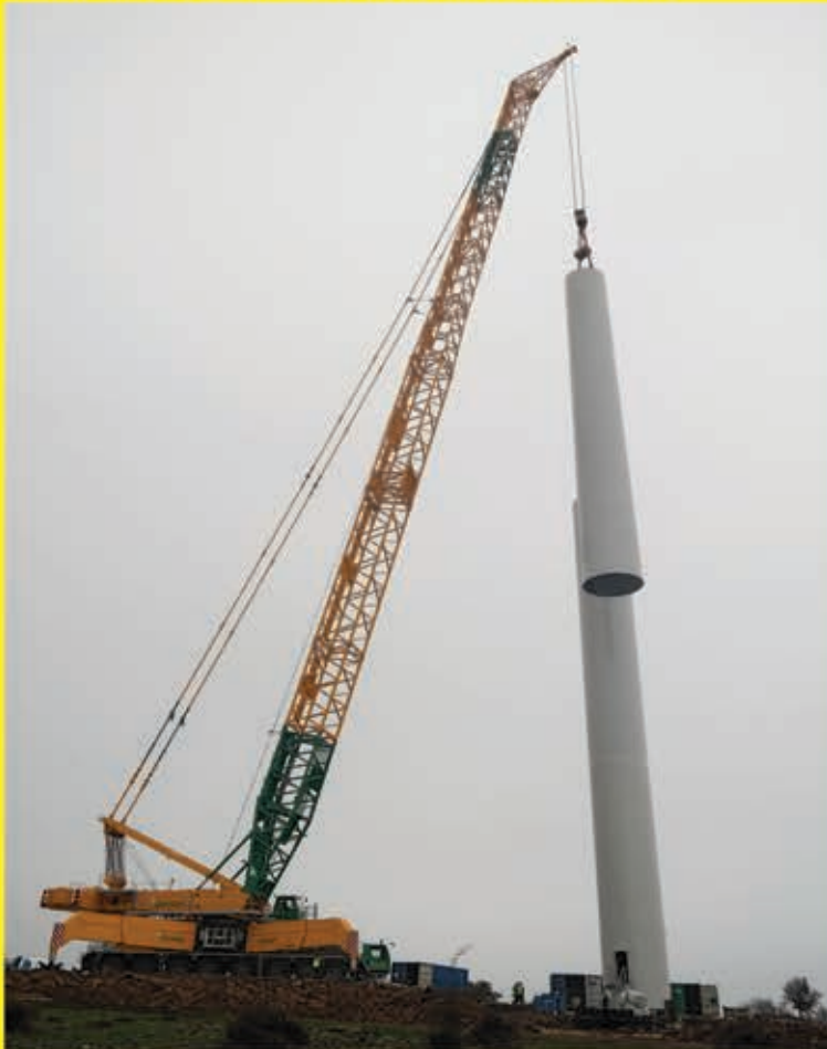
Installation of wind turbine by Liebherr LG 1750 at Enez / Edirne.
