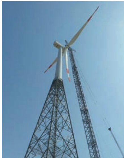
Liebherr LR 1600 lattice boom crawler crane working for Suzlon at the Naliya site erecting wind turbines with hybrid lattice and closed section towers with 120 metre hub height
