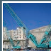
KOBELCO SL6000, 550 ton capacity
