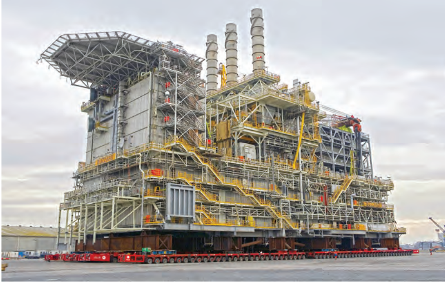
A 13,300 tonne offshore platform on Scheuerle SPMT
