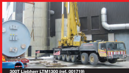
300T Liebherr LTM1300 (ref. 001719)
