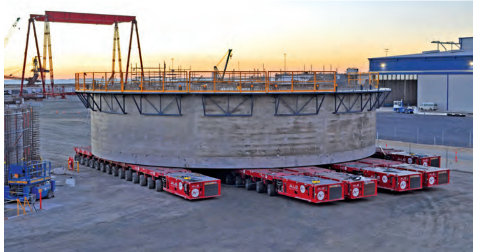
ALE transporting a concrete element on 84 axle lines of Scheuerle SPMT
