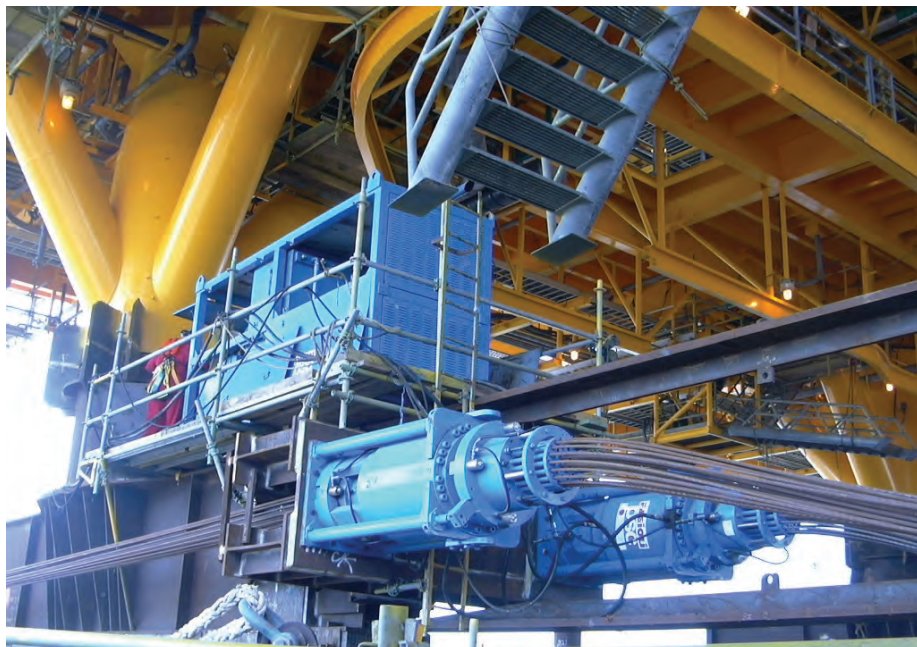
Strand jacks in operation being used for horizontal movement rather than vertical lifting
