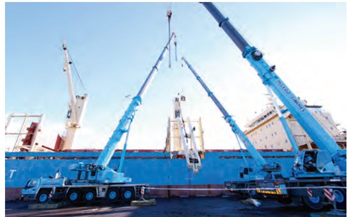
Three Grove all terrain cranes salvage a collapsed boom on a ship crane
