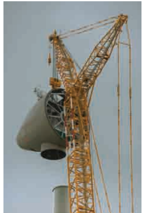
The 170 tonne nacelle is lifted at a radius of 40 metres
