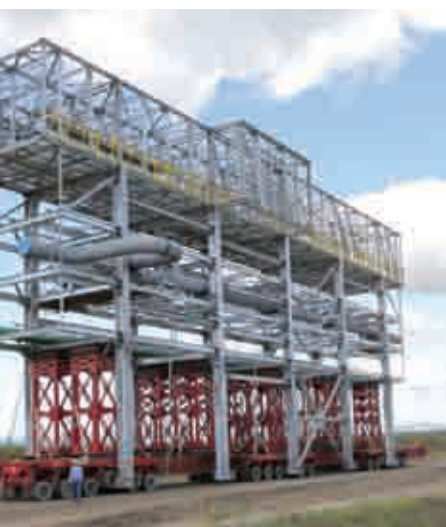
Transdata use SPMT to transport a pipe rack internal haulage at a petrochemical facility in Rio de Janeiro, Brazil
