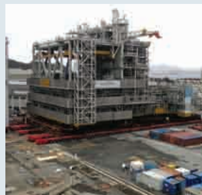
The weights of the various modules ranged from 1,600 to 11,500 tonnes
