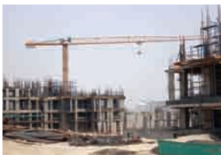
Liebherr's 85 EC-B 5i tower crane is designed for confined sites. The tower sections have a footprint of 1.2 m x 1.2 m
