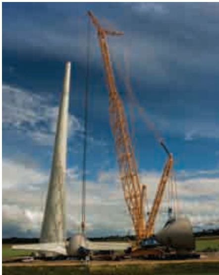
Once the turbine towers had been assembled, the CC 8800-1 was used to lift the remaining parts of the turbine into position
