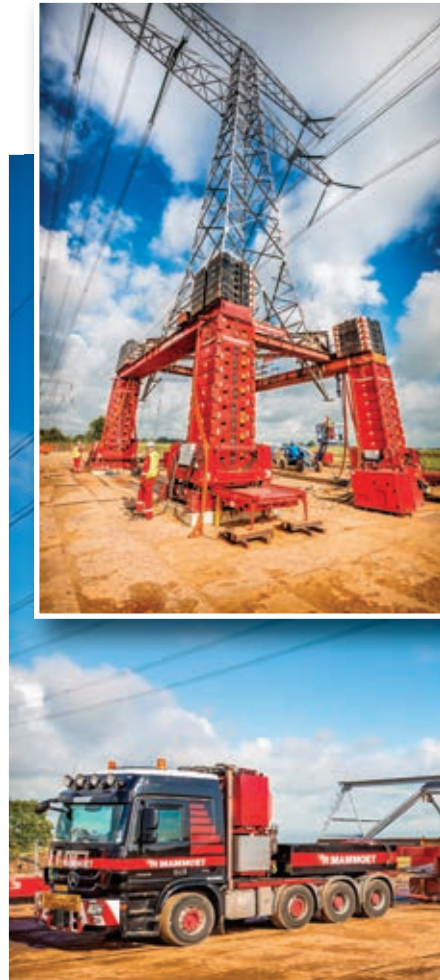
The power pylon had to be elevated by four metres in situ, while maintaining a live power supply
