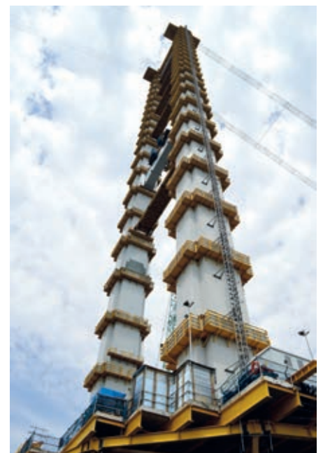
The towers have already reached a height of 252 metres and catwalks and platform decks are being laid from the north and south ends
