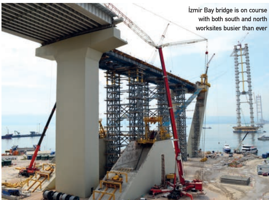
The towers have already reached a height of 252 metres and catwalks and platform decks are being laid from the north and south ends
