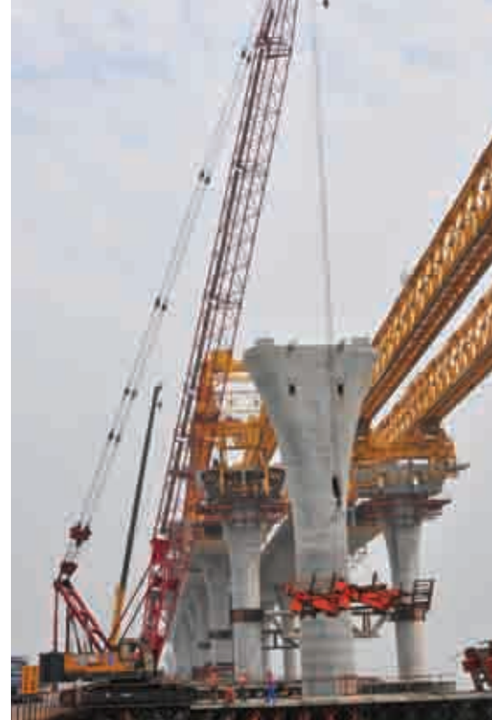
A Sany SCC1000C lifting a section of the Jiashao Cross-Sea Bridge in Hangzhou Bay, Shaoxing, China
