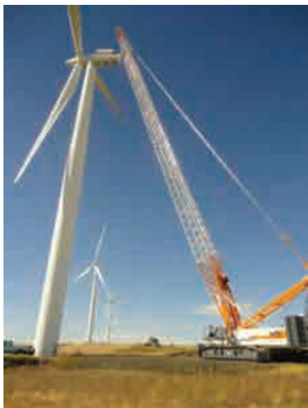
A Zoomlion QUY260 crawler crane owned by Axis Crane helps install wind turbines at a wind farm in the USA
