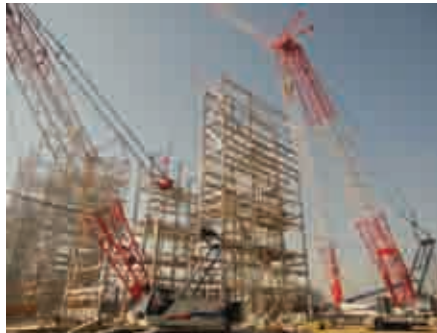
A Zoomlion QUY260 crawler crane at work at the Reliance Sasan Power Station in Varanasi, India
