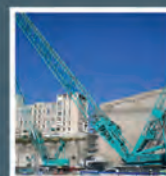
Kobelco SL6000, 550 ton capacity
