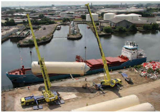
Lifting the last vessel from the hold
