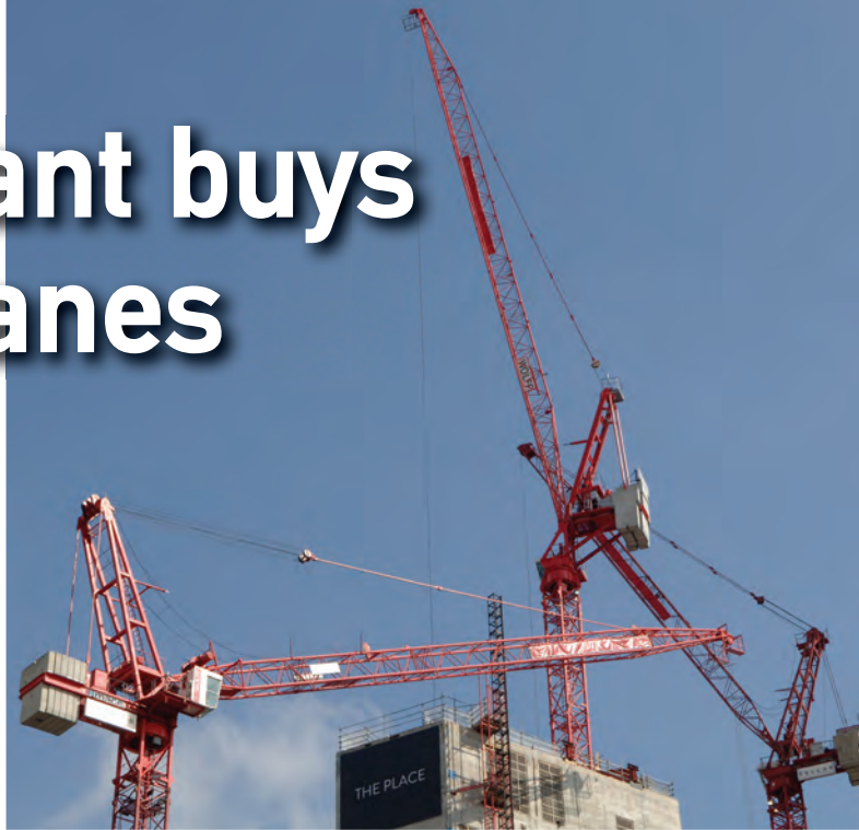
HTC Plant Wolff tower cranes on The Place project in London
