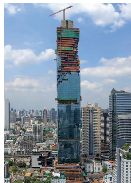
The 21LC290 flat top working on top of the MahaNakhon tower (IMAGE: PACE DEVELOPMENT CORPORATION)
