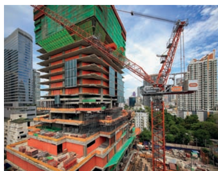
Close view of the LCL310 24t luffer at the MahaNakhon project (IMAGE: PACE DEVELOPMENT CORPORATION)
