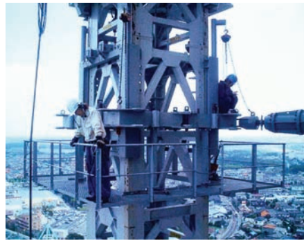
Fixing the tie-in beams using the work platform
