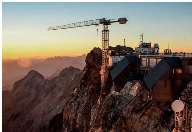
The Liebherr 150 EC-B flat top crane on the Zugspitze
