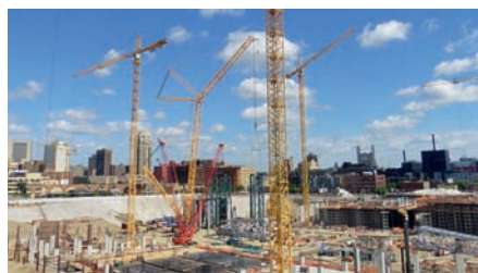
Liebherr towers from Morrow Equipment at the Minnesota Vikings stadium project in the USA
