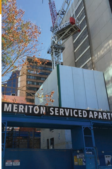
Jaso J280 PA.2R rigged on the lift shaft climbing system on a cramped city site in Sydney, Australia
