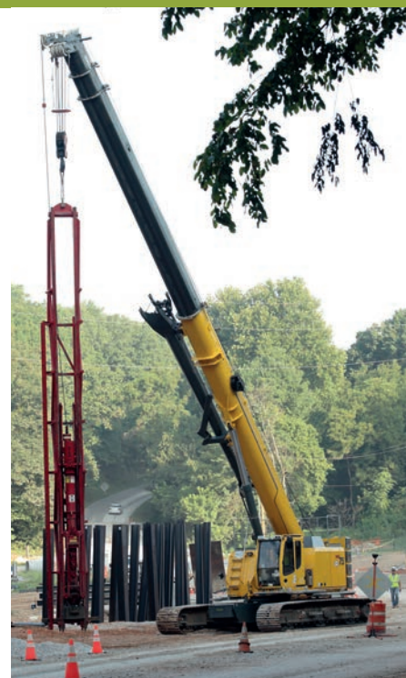
This Grove GHC75 was used as a pile driver in tough conditions, driving piles into the wet, uneven soil of a creek bed with only a 30-foot (10 metre) radius for contractors to work in
