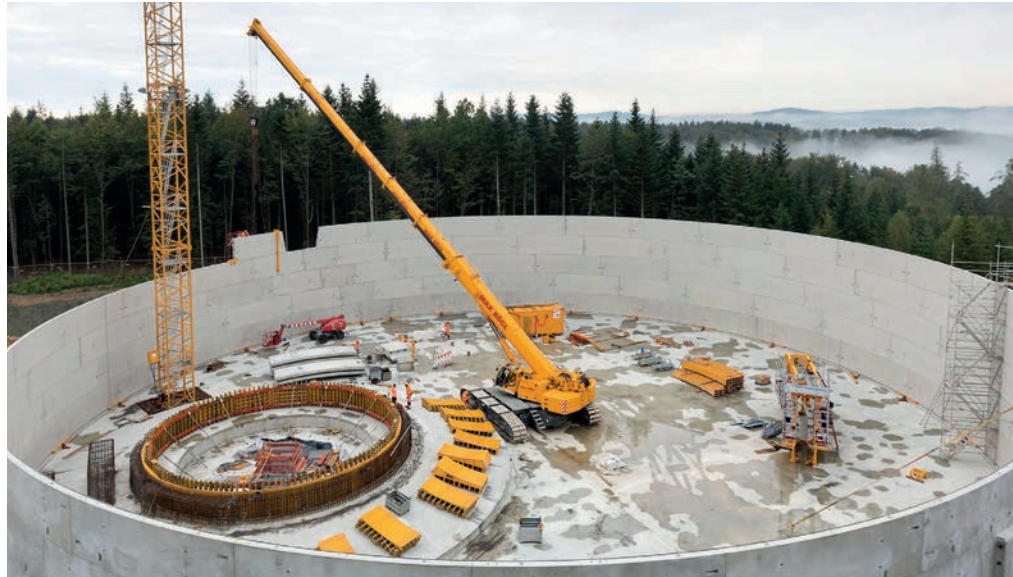
From its central position the Liebherr telescopic crawler crane can reach every point of the 15 metre reinforced concrete wall. Once built, the telecrawler will be lifted out of the structure
