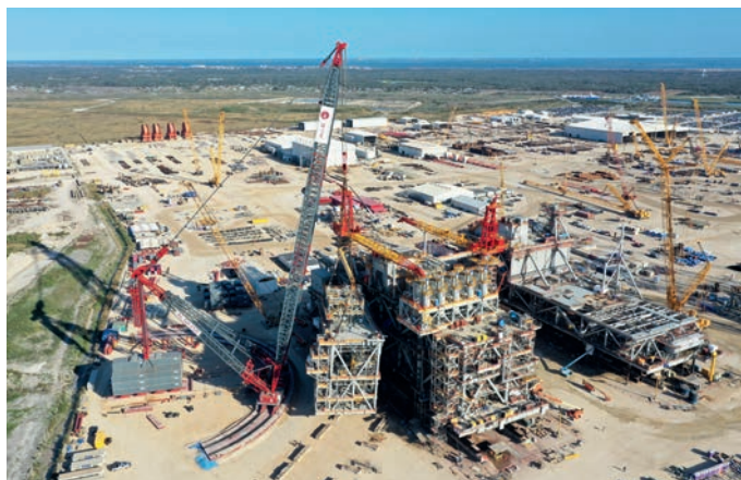
AL.SK350 with close to 3,000 tonnes on the hook at Ingleside, Texas, USA
