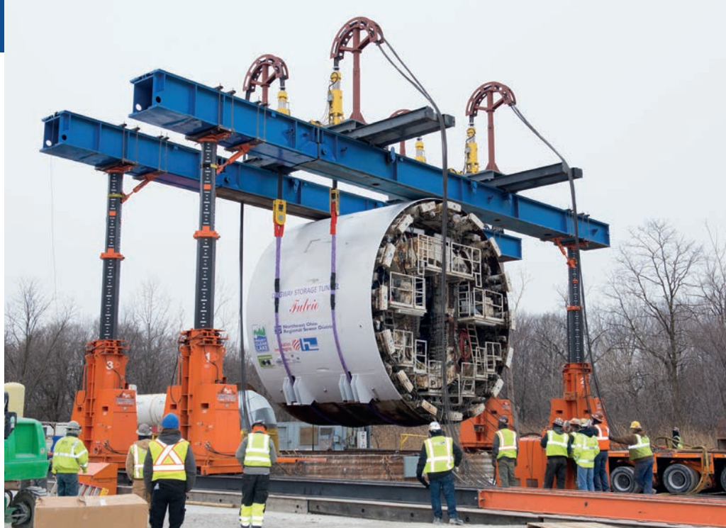
Cortland Company slings were used to lift a 500 tonne tunnel boring machine in Ohio, USA
