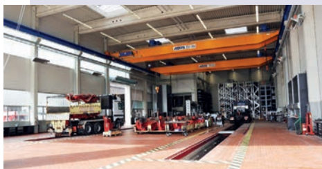
The 2,500 m 2 servicing workshop in Bavaria
