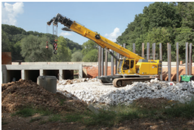
The GHC75's expandable, heavy-duty crawler tracks eliminated the need for deploying outriggers, which enabled the crane to maneuver in tight quarters over wet, uneven terrain.
