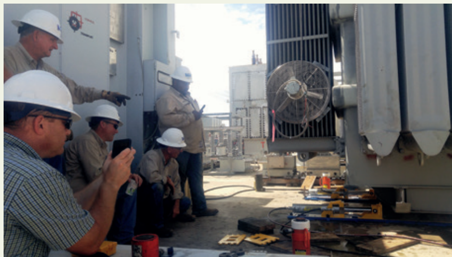
Lower Colorado River Authority's riggers are immersed in training on a Hydra-Slide XLP150 skidding system, moving a transformer in the yard.
