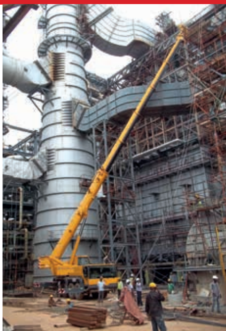
A 70 tonne capacity Liebherr LTM 1070 wheeled mobile crane belonging to Bilfinger Neo Structo working at the BPCL refinery expansion project
