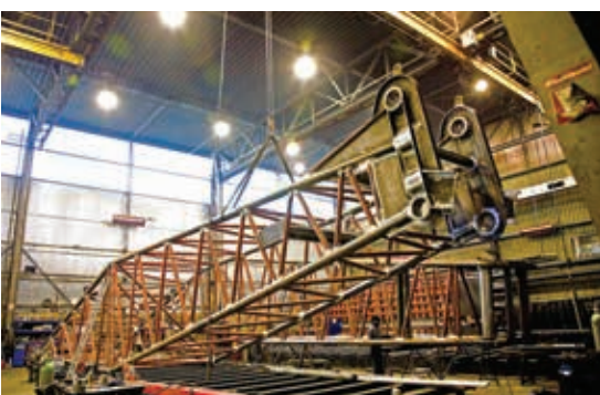
Repair and refurbishment at Avezaat
