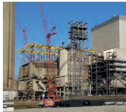
Maxim cranes are assisting in the tear out and replacement of a precipitator and a boiler.
