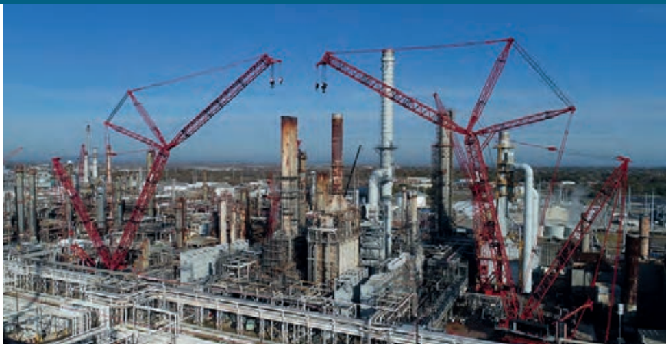
Maxim cranes are assisting in the tear out and replacement of a precipitator and a boiler.
