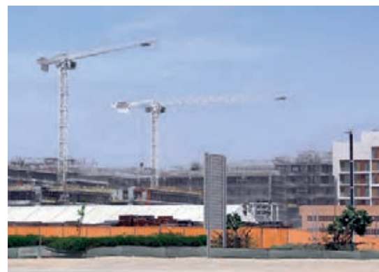
Six Construct is using two Potain MDT 259 J12 CCSs to help build a residential complex in Abu Dhabi
