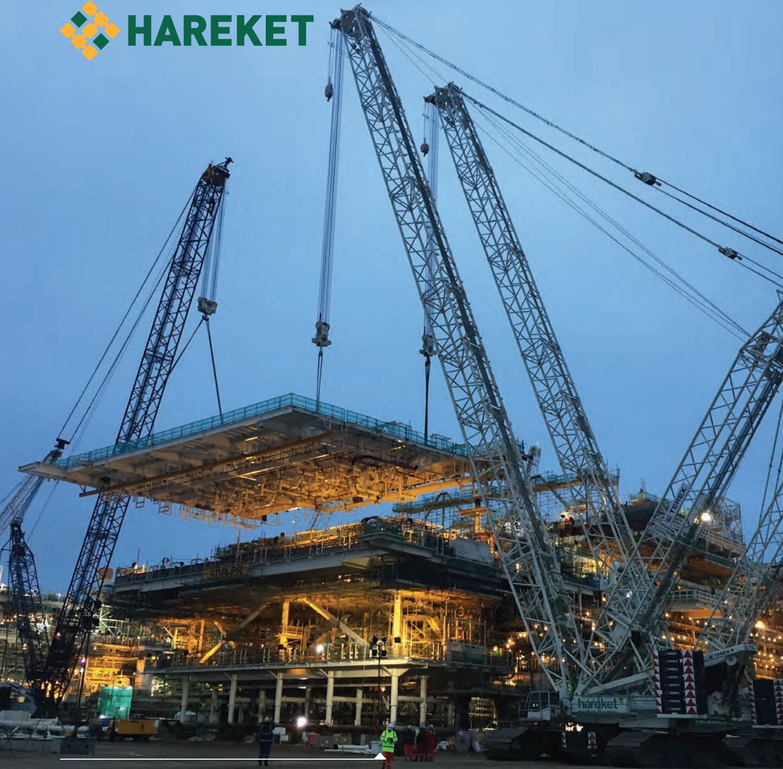
Heavy lifting operation of 392 tons Upper Deck Panel with 3 units 600 tons capacity crawler cranes.
