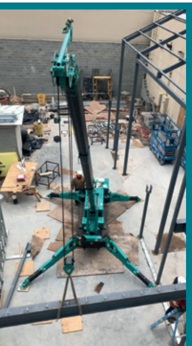
Austin Iron recently used a Maeda MC305-2 for a steel erection project. With its 51-inch body width, 6,560 pound maximum capacity and 47-foot maximum lift height, the Maeda MC305-2 helped the Texas company complete its project within a limited construction space.
