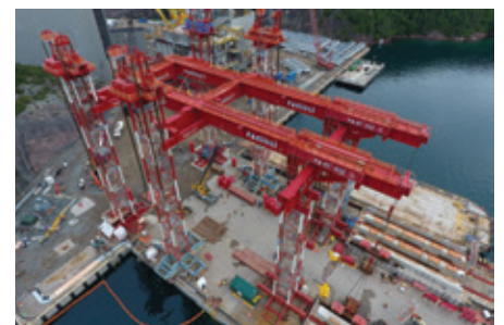
Fagioli assembled and installed modules into a topside unit on a customized pier.
