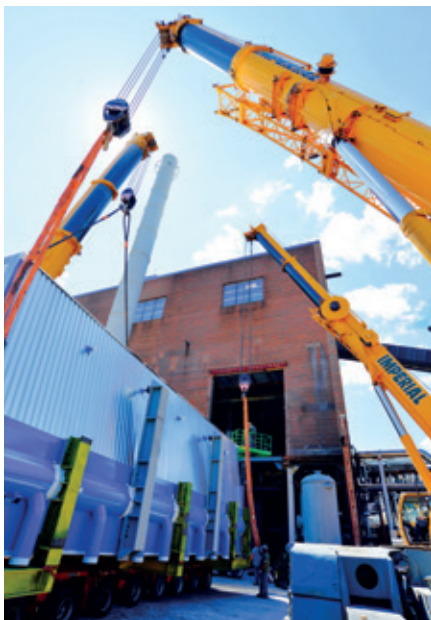
The boiler was removed from Bay Crane's 10-axle Goldhofer THP/CA trailer onto a Goldhofer SPMT so it could be moved through the plant.
