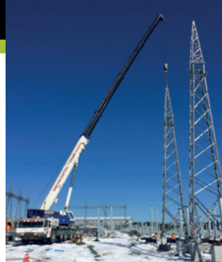
PHOTO: CAPITAL CRANE
