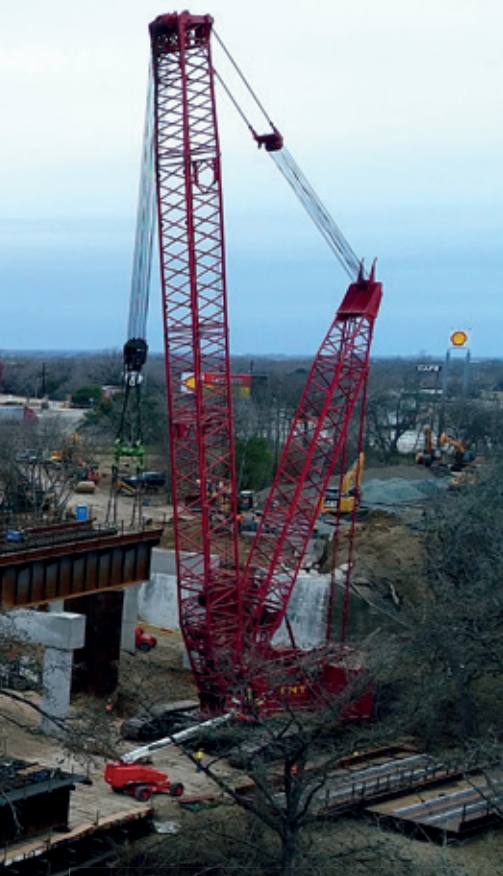
Ground preparation was critical to the lifts and required a significant layer of rock and then wood and steel pads.
