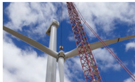
Mammoet installing the last of 75 rotors at the Ararat Wind Farm in Australia
