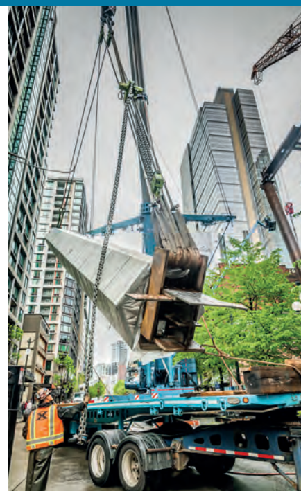
The rigging plan allowed single crane picks where possible and didn't require the use of a tailing device.
