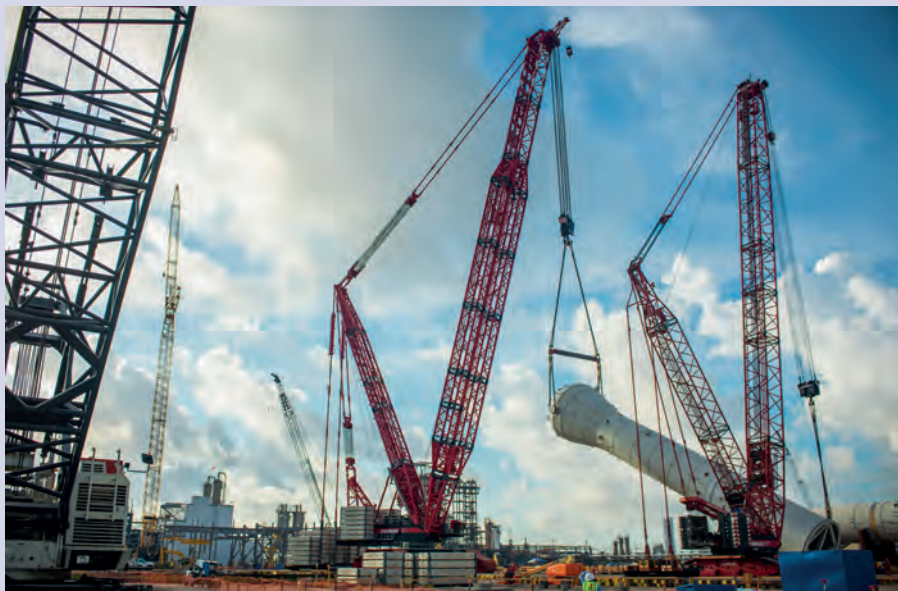
With its massive boom rising high into the sky, the Liebherr LR13000 was strategically placed to lift and install both reactors from one position. The Terex CC2800 handled the tailing work.
