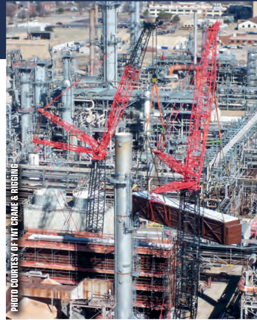
TNT Crane & Rigging rigged its two Liebherr LR 1350 crawlers with a complicated system of spreader bars, chain falls and slings to lift a 425,000-pound convection section of a crude heater at a refinery in Ponca City, OK.
