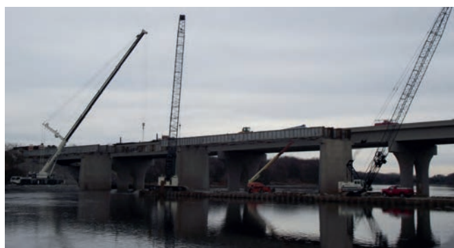
Two Terex crawlers and an AT work at the Highway 24 bridge.
