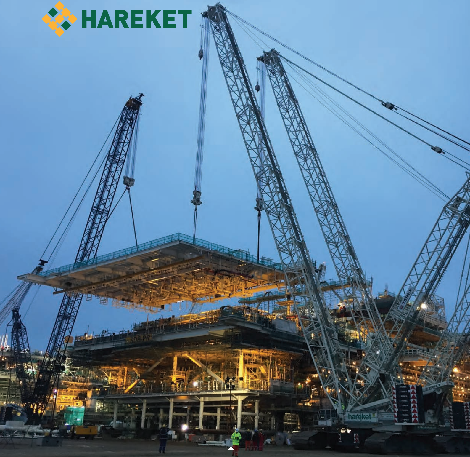
Heavy lifting operation of 392 tons Upper Deck Panel with 3 units 600 tons capacity crawler cranes.
