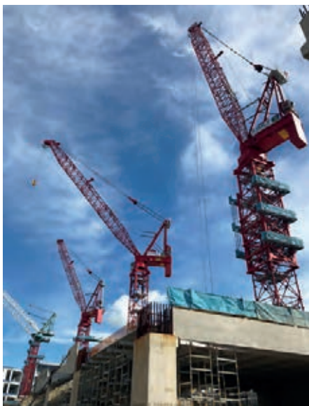
After minor modifications of the upper crane design, reducing the number of falls and replacing the boom nose with a standard jib end section for two fall operation, the Krøll K1650L becomes a versatile heavy lifter for precast concrete construction in Singapore
