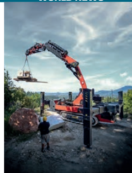
The Palfinger Crawler Crane type PCC 115.002 in action
