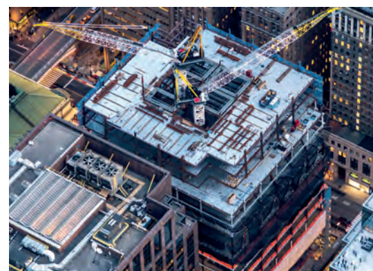
Two custom-built Favelle Favco M760Ds with reduced tail radius of 7.63 m to fit into the concrete core of the One Vanderbilt project in New York, USA
