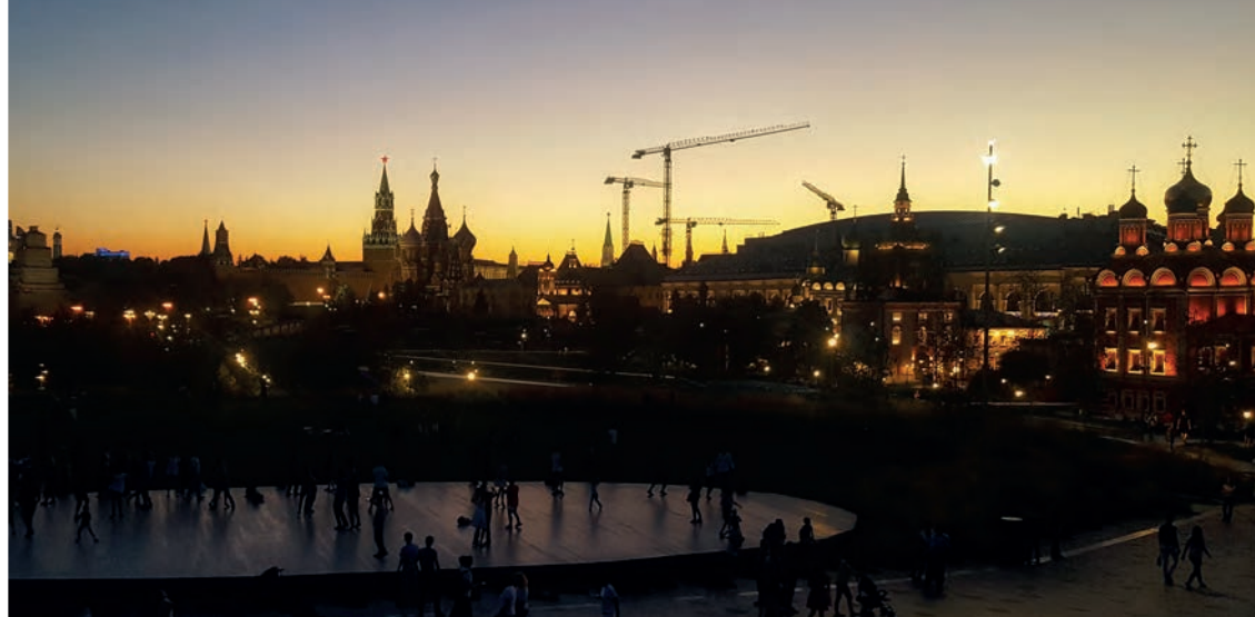
Four flat top cranes from Comansa working in Red Square, Moscow, Russia, near St. Basil Cathedral. The photo was taken by the Spanish tower crane manufacturer's area sales manager for Russia, Greg Teyf.
