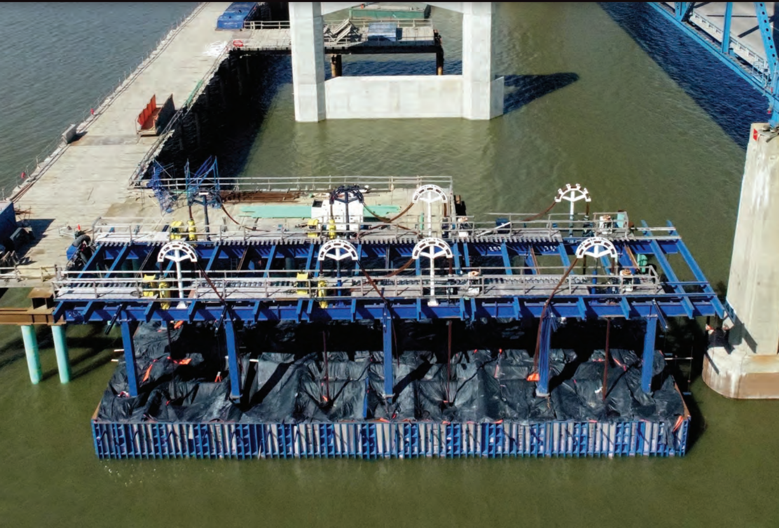
8 HSL2000 STRAND JACKS USED DURING CONSTRUCTION OF BRIDGE FOUNDATION. PHOTO CREDIT: MCCLUGAGEBRIDGE.COM
