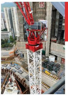
WOLFF Boost, anti-collision interface, fine driving modes, automatic performance optimization for the trolley and hoist as well as the WOLFF Link remote maintenance system with real-time display of the crane display.
